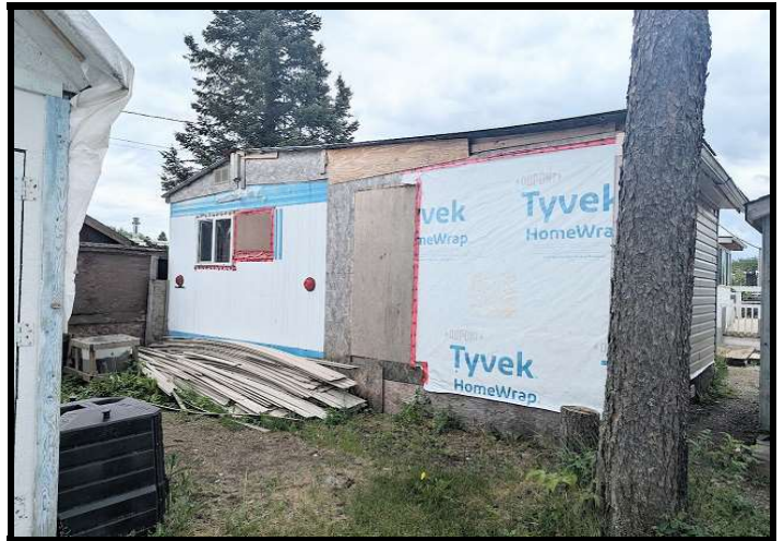
Back of Home & extra siding to finish
