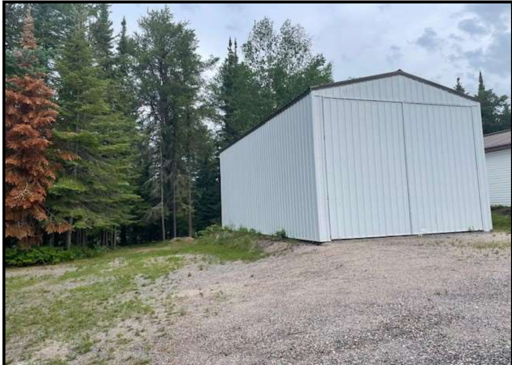
20'5" x 36' Metal Storage/Shop
