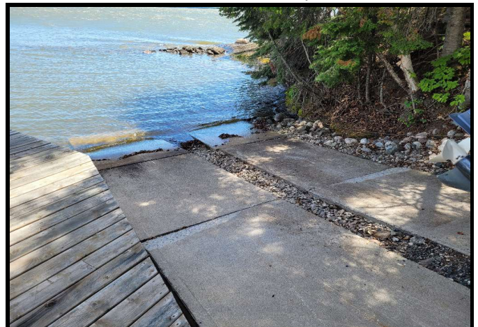
Sheltered access with concrete pad boat launch
