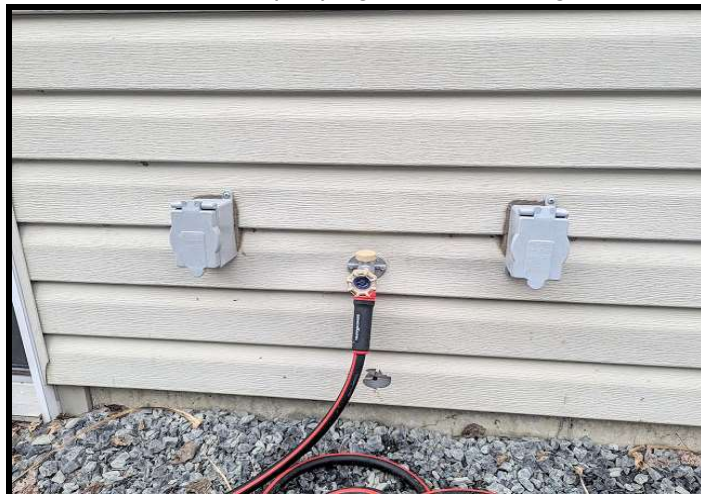
30&50 volt camper plug,can be used together
