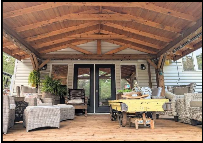
Stunning Timber-Frame Roof
