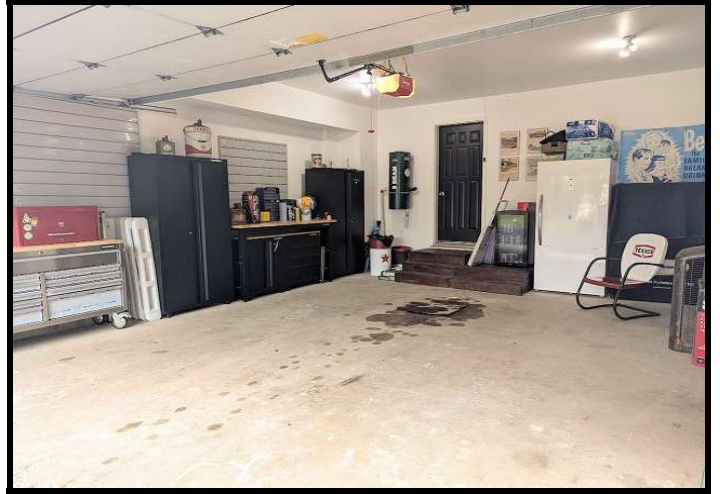
Newly Drywalled Garage Interior
