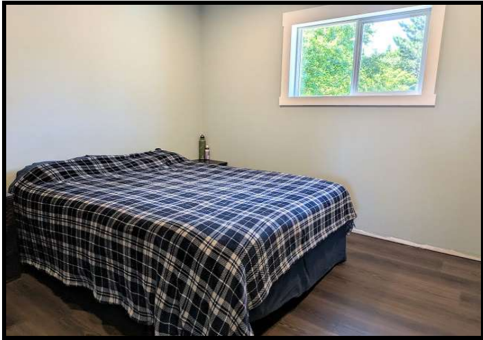
Primary Bedroom, new flooring, drywall & lighting
