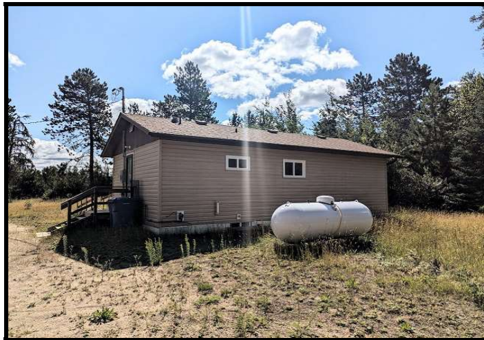
Rear of Home, rental propane tank
