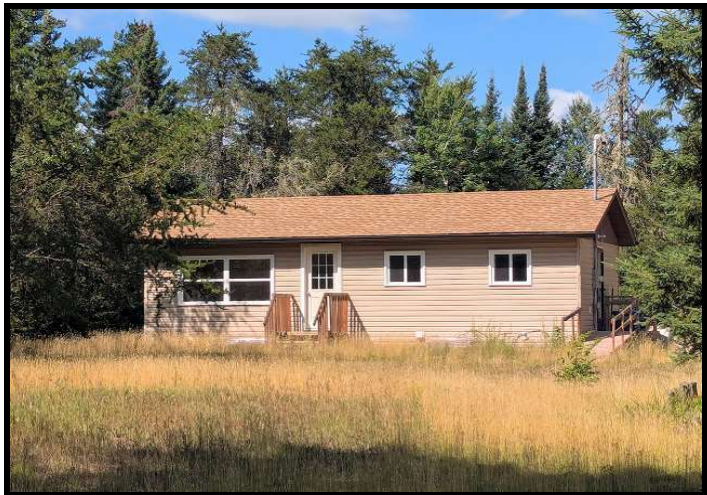
Shingles & Vinyl Siding replaced in 2016
