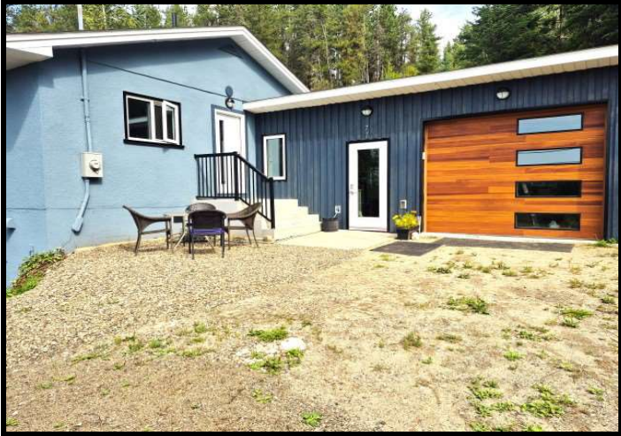
Attached Garage with 100 amp service
